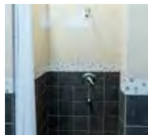
REST ROOM & SHOWER
